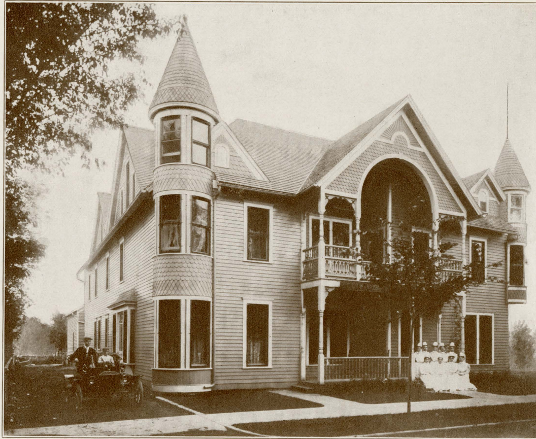
SOUTHWESTERN MINNESOTA HOSPITAL, HERON LAKE, MINN. (North Side)
